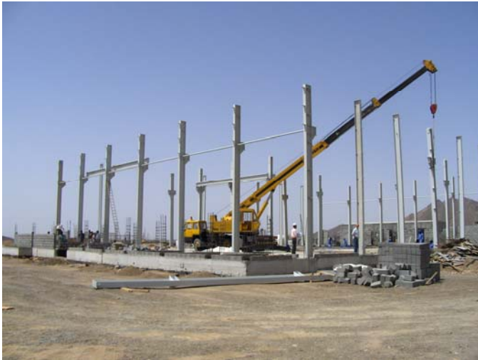
Top: The initial steel girders been positioned
